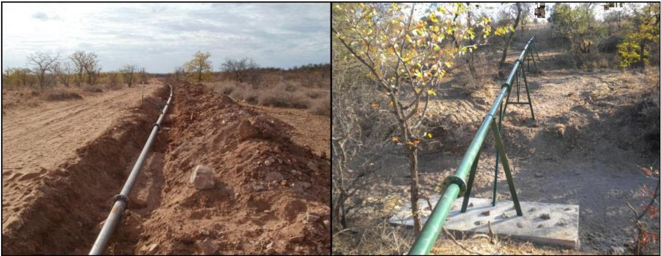
**Figure 18-10 Water Pipeline and Crossing**
