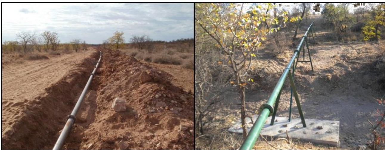
**Figure 18-10 Water Pipeline and Crossing**
